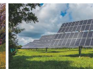
Solar Pumping System
